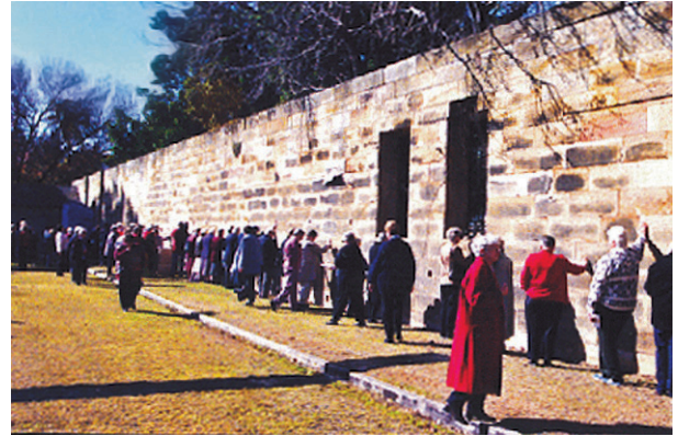
Sisters of Charity at the last remaining wall of the Factory, 2005. Photo by Bruce W. Stephens.
