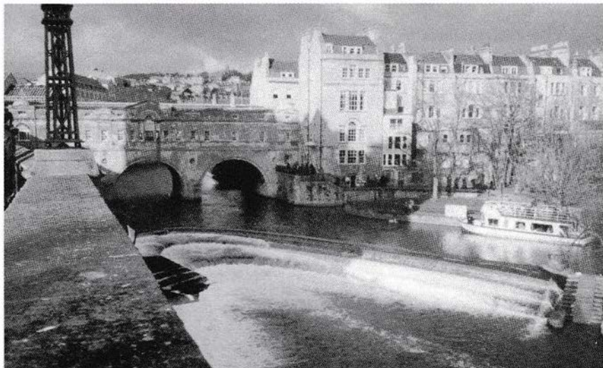
The renowned Scottish architect Robert Adam designed the Pulteney Bridge in 1770 based on the Ponte Vecchio of Florence. Beneath the bridge flows the River Avon over the graceful weir.
